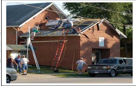
Operative Lodge Roof Installation
